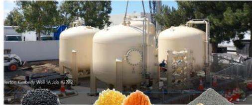
Granular Activated Carbon (GAC)    Ion Exchange (IX) Resin    Alternative Adsorbents (AA)
