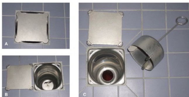
Figure 1. Shower drain design. The whole installation is covered by a heavy stainless steel lid (A), which is designed to discourage patients from opening and to prevent accidental removal. The drain (B) is designed to be wide, so it can be easily cleaned and disinfected. A bubble cap insert (C) prevents odors and splashing and can be removed for sterilization.
