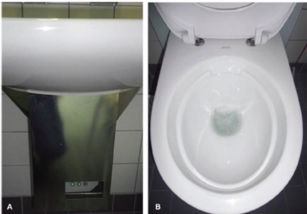
Figure 2. Hygiene siphon and rimless toilet. The Hygiene siphon uses vibration (50–200 Hz), high temperatures (85°C), and ultraviolet light to prevent biofilm formation. It is covered to discourage a frequent change of settings and for cleaning and disinfection purposes.
